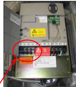
PICTURE 13: Single-Phase Motor Inverter Box
