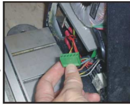
Cable Connector (Right Gantry Leg)
